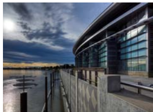
Freeport Regional Water Project (EBMUD and Sacramento County)
