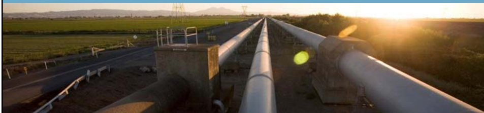
EBMUD Mokelumne Aqueduct
