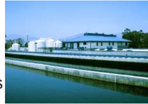
City of San Diego Otay Water Treatment Plant
